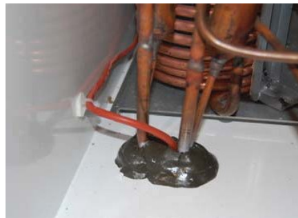
Introduction of the sensor from the top of the engine compartment
